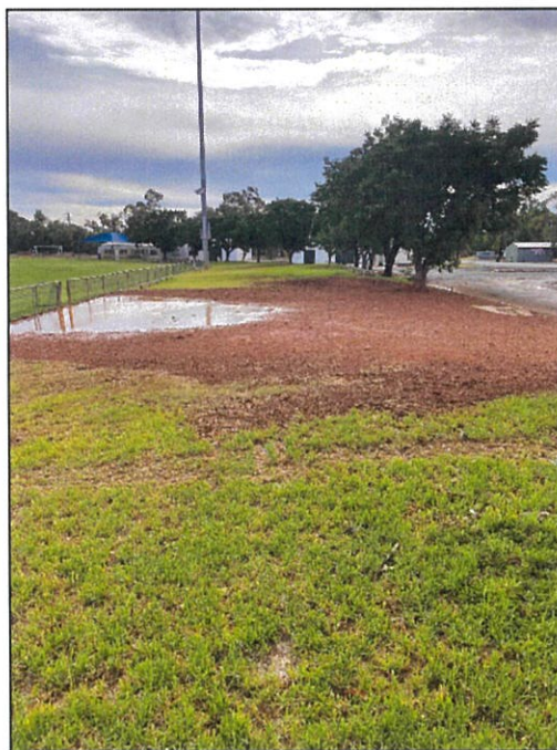
Former grandstand upon completion of lead paint removal and demolition works, visual inspection and soil validation sampling.
