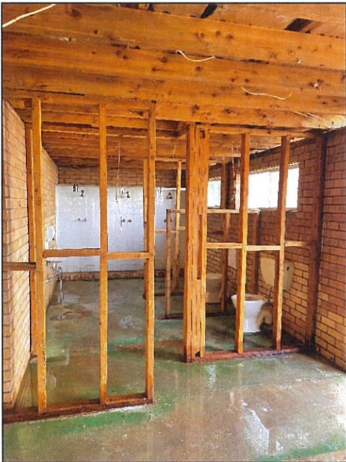
Internal male bathroom walls and ceiling upon completion of visual clearance inspection.
