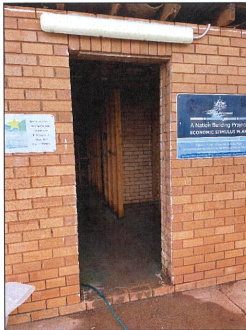
External fascia and guttering upon completion of lead paint removal works, visual inspection and baseline soil sampling.
