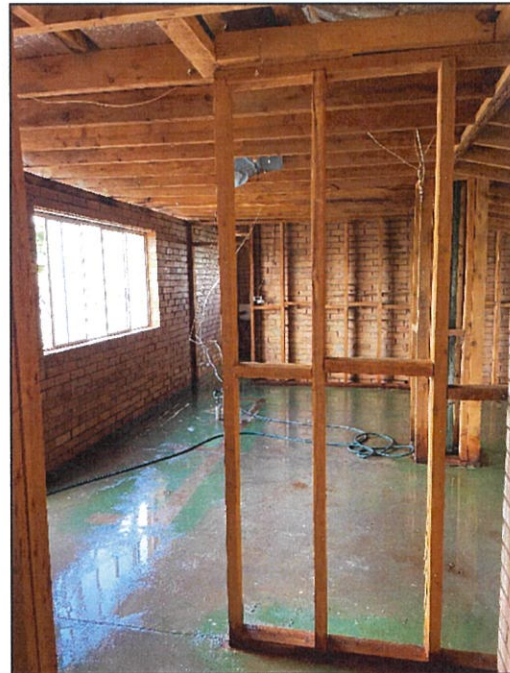
Internal main room walls and ceiling upon completion of visual clearance inspection.
