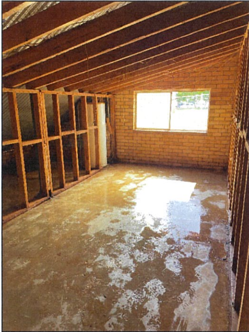
Internal kitchen walls, ceiling and floor upon completion of visual clearance inspection.
