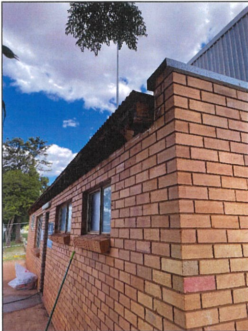
External eaves upon completion of visual clearance inspection.
