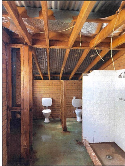
Internal female bathroom walls and ceiling upon completion of visual clearance inspection.
